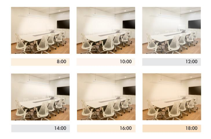
With human centric lighting function, color temperature and brightness will change automatically according to the time of the day. End-user can easily choose pre-programed curve or customize their own curve profile via Koolmesh Bluetooth APP, with a CCT change from 2700K to 6500K.
